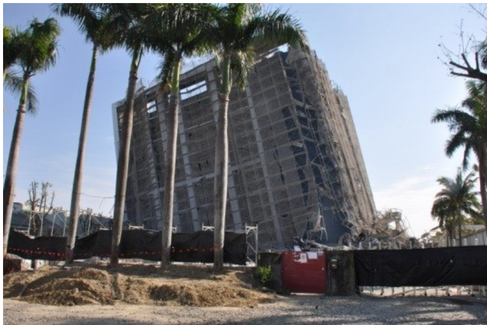
(a) Severe tilt failure (New Wanglin Building, Tainan, Taiwan) (Hsu and Ho, 2016).
