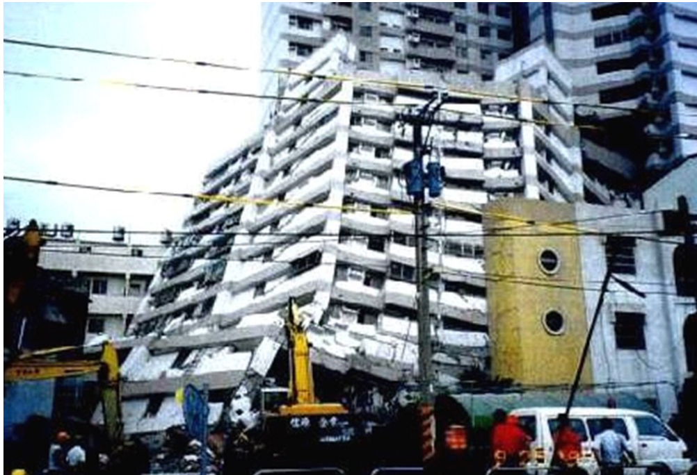
(a) Tilt and fall failure (Taiwan Yunlin Fugui Mingmen Building).
