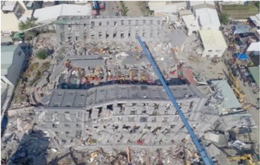
(b) Overturning failure (Weiguan Building, Tainan, Taiwan).
